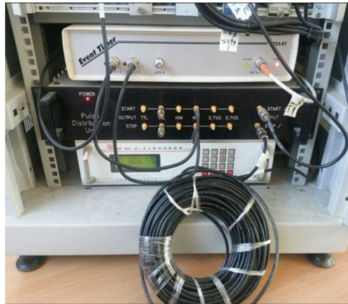
Fig.6 30m cable added to A033-B
